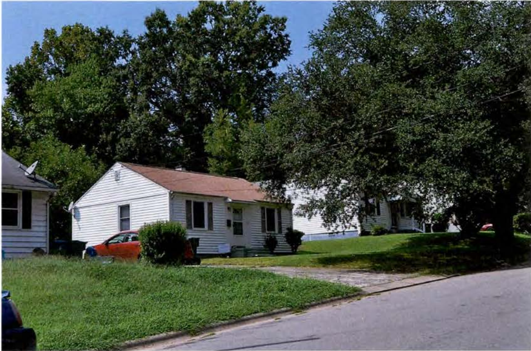
1208 and 1206 Rosewood Street
