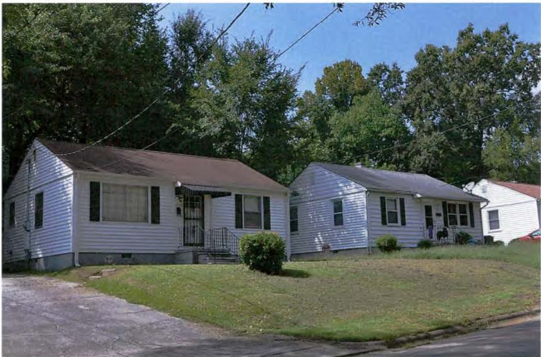
1212 and 1210 Rosewood Street
