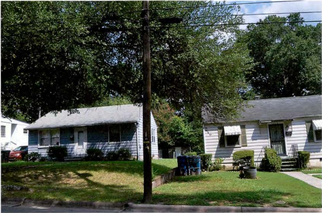
1213 and 1215 Rosewood Street
