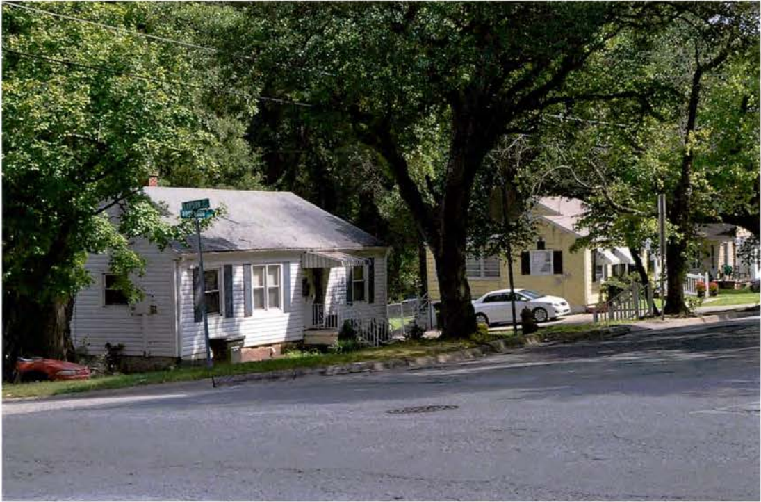
1301 and 1303 Rosewood Street
